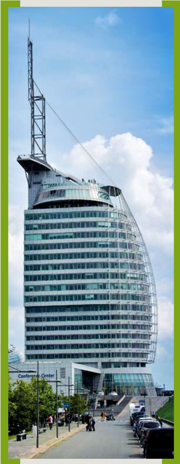
The Sail City building in Bremerhaven
